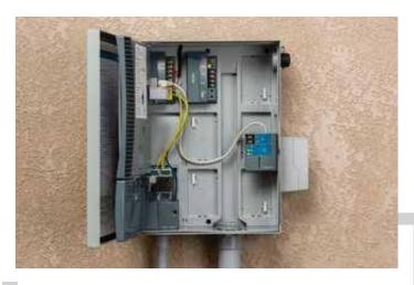
Installing a commercial controller is challenging without an internet connection. So what can contractors do when local Wi-Fi or LAN access is out of range or unavailable, or they aren't allowed to log in to their customers' secure network? Use the ICC2 Cellular Connection Module.
